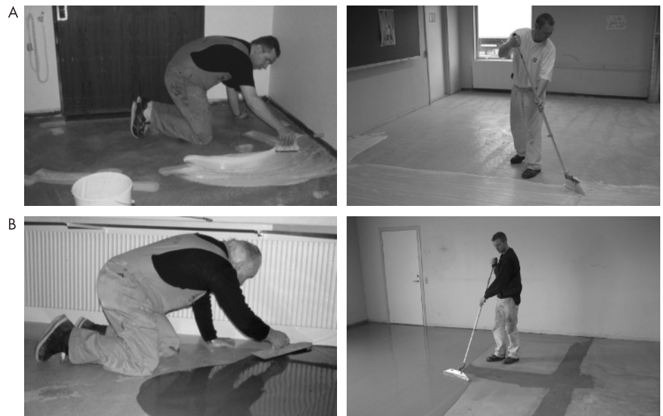
Figure 2 (A) Floor layers. Gluing; working traditionally (left), and using new (right) working methods. (B) Floor layers. Filling; working traditionally (left), and using new (right) working methods.
