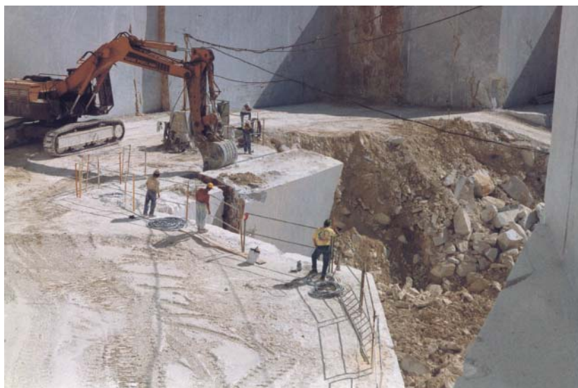
Figure 2 Overturning of the bench with an excavator.
