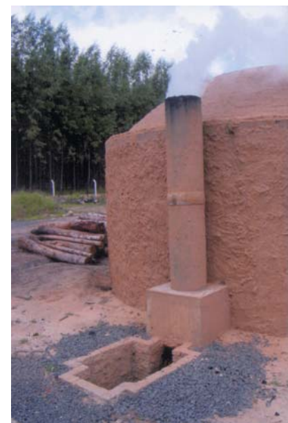
Figure 8 A kiln that enables starting fire from the bottom.
