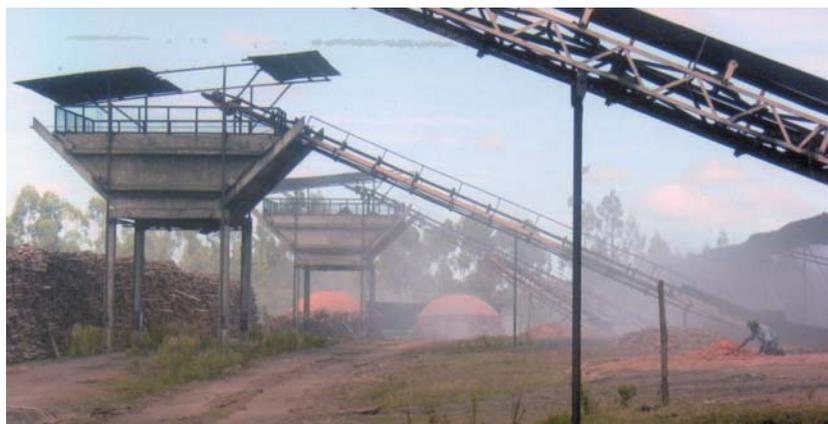
**Figure 7** Silos that enable direct charcoal truck loading.
