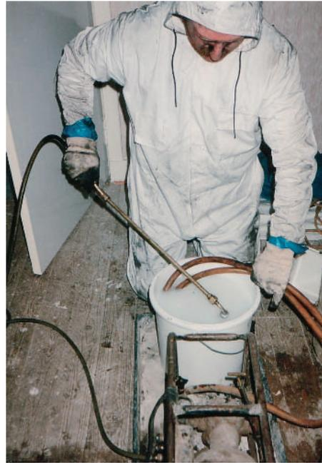
**Figure 2** Worker in coverall washing spray lance.
