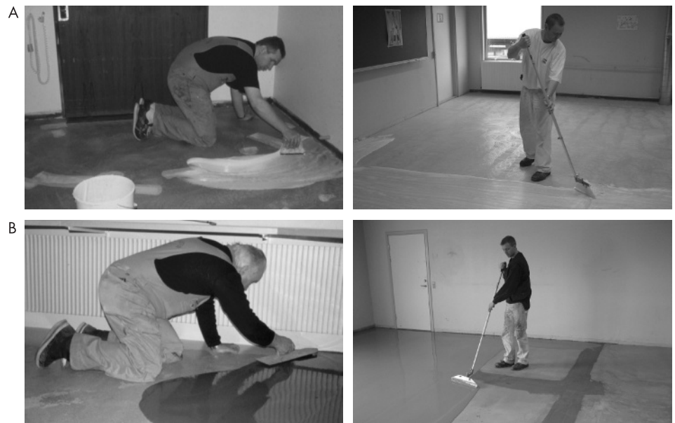
Figure 2 (A) Floor layers. Gluing; working traditionally (left), and using new (right) working methods. (B) Floor layers. Filling; working traditionally (left), and using new (right) working methods.
